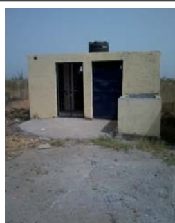
Picture 4: Toilet in Chavaj PS, Bharuch (29.05.2013)
